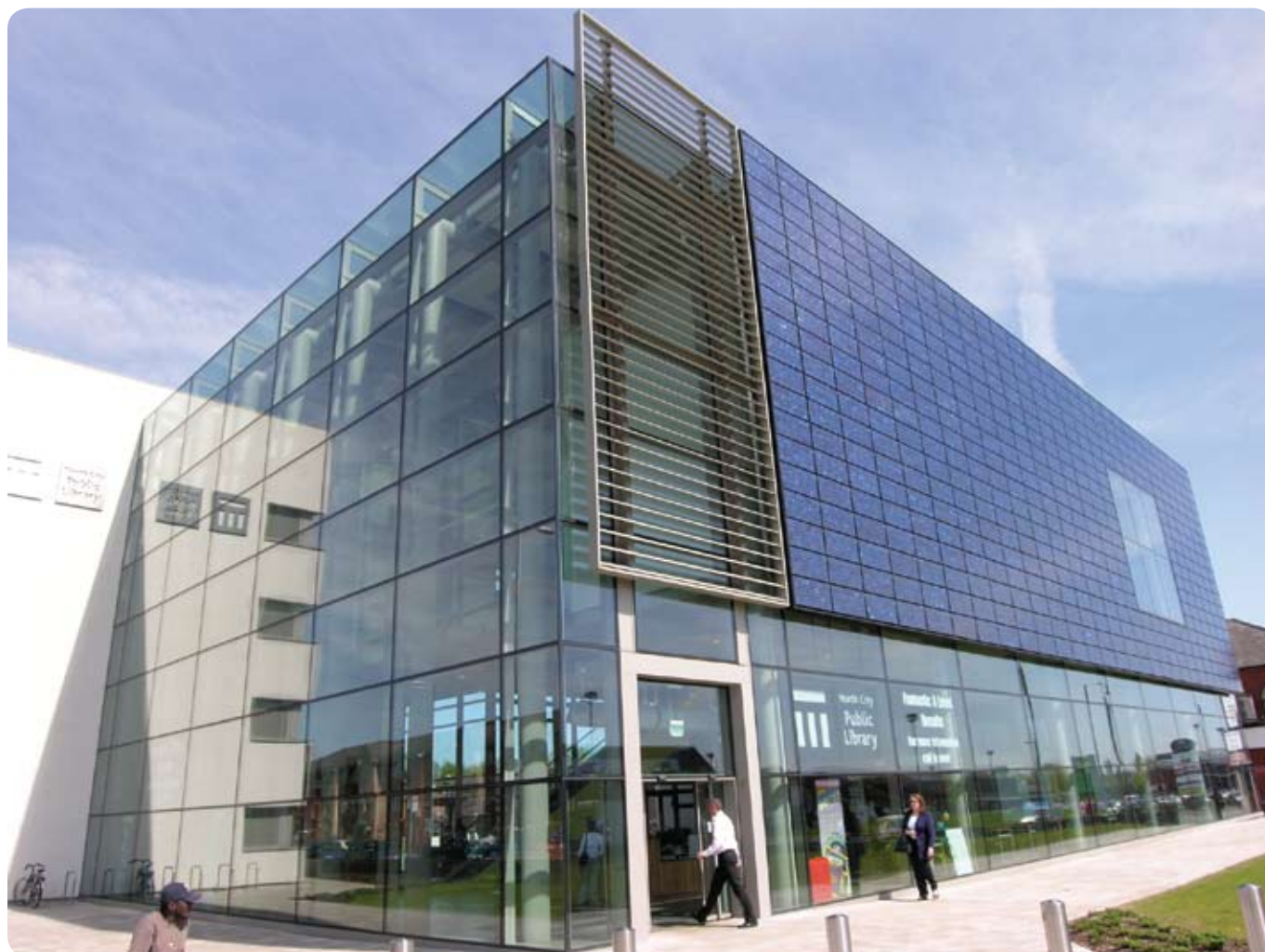
Solar facade, Manchester College of Art & Technology
