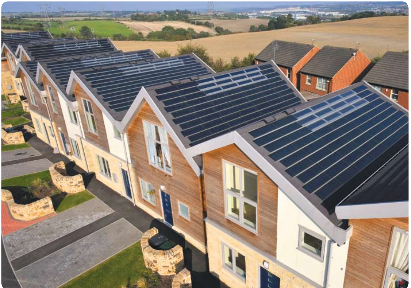
Solar roofs, Rothham, South Yorkshire
