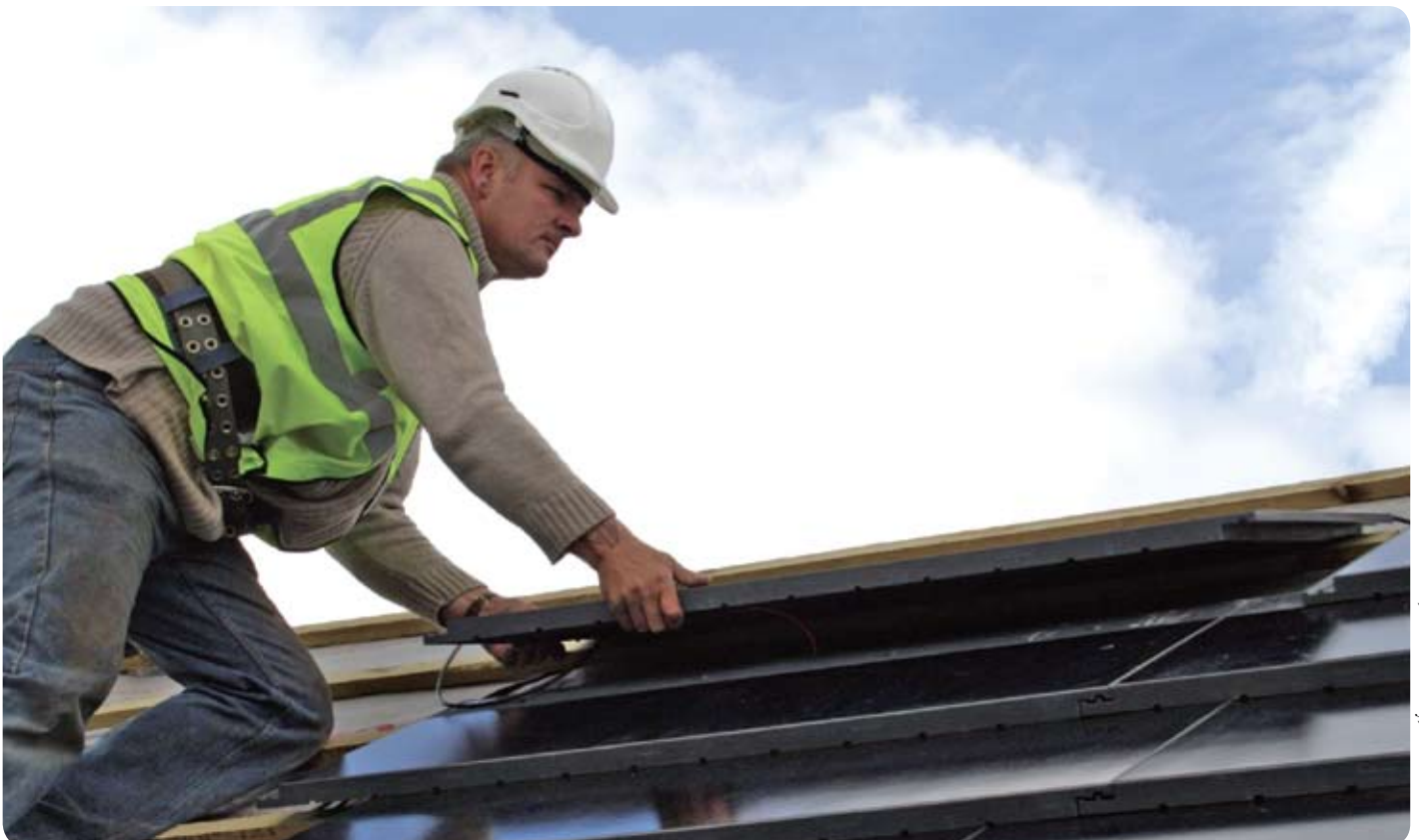
Solar roof tile installation, Melton Mowbray, Leicestershire
